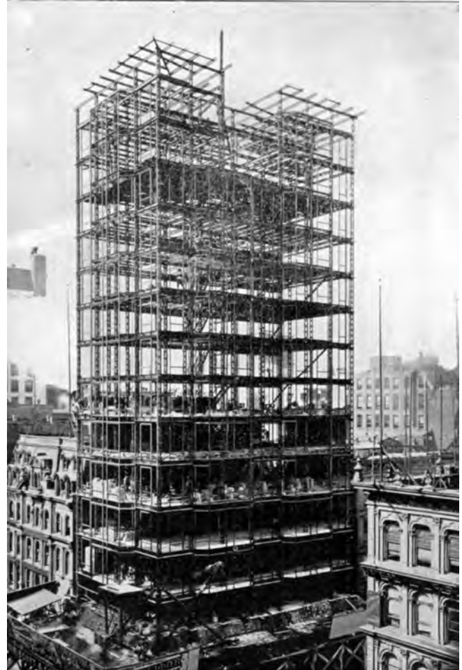
The Reliance building being built in approximately 1890.
